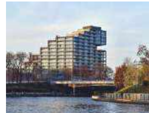
FA 50N HI, TM 62HI NORDIC HAVEN - RESIDENTIAL BUILDING NORDIC HAVEN BYDGOSZCZ / BYDGOSZCZ 53
