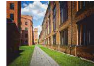
FA 50N, TM 62HI INDUSTRIAL SCHEIBLER'S LOFTS LOFTY SCHEIBLERA LODZ / ŁÓDŹ 61
