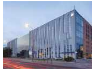
FA 50N OFFICE BUILDING - W.M. LEGNICKA PARK BIUROWIEC - W.M. LEGNICKA PARK WROCLAW / WROCLAW 22
